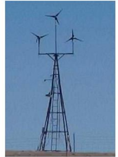
d. Three rotor Array Wind Turbine
