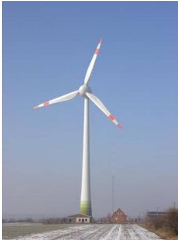
4.5 MW Wind turbine 112 m dia.
