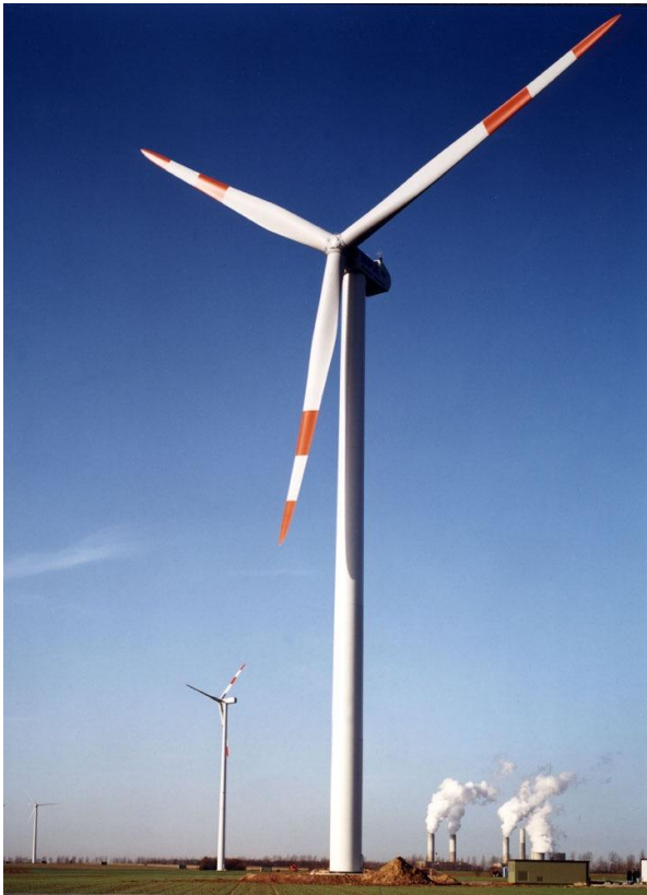
2.5 MW Wind turbine 80 m dia.
