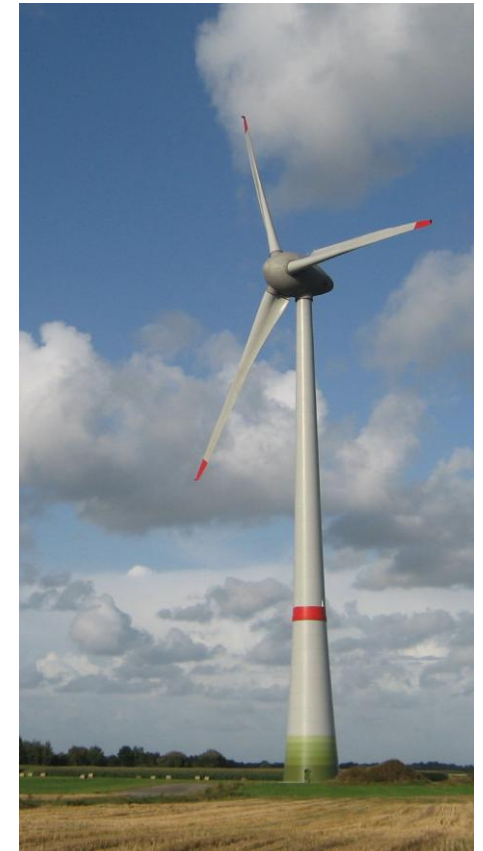
7.5 MW Wind turbine 126 m dia.
